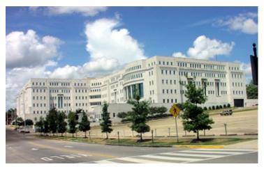
The Gordon Persons Building is a six floor, 60,000 square foot state government office building in Montgomery Alabama making this build the second largest State Building in Alabama. The structural design concept of the Persons Building included placement of concrete columns down the center of its main corridors. The small pagodas in the foreground house stair exits from the pedestrian tunnel which runs under Union Street and connects the
